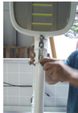
Use No.14 trigger to fix the lamp screw
