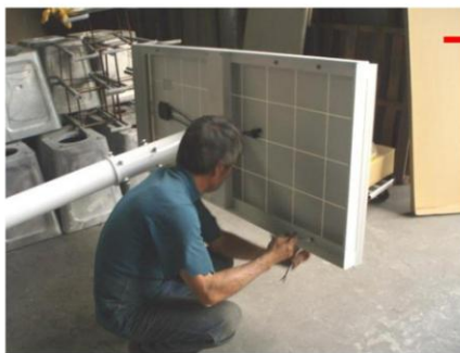
Install Solar Panel and Cable
