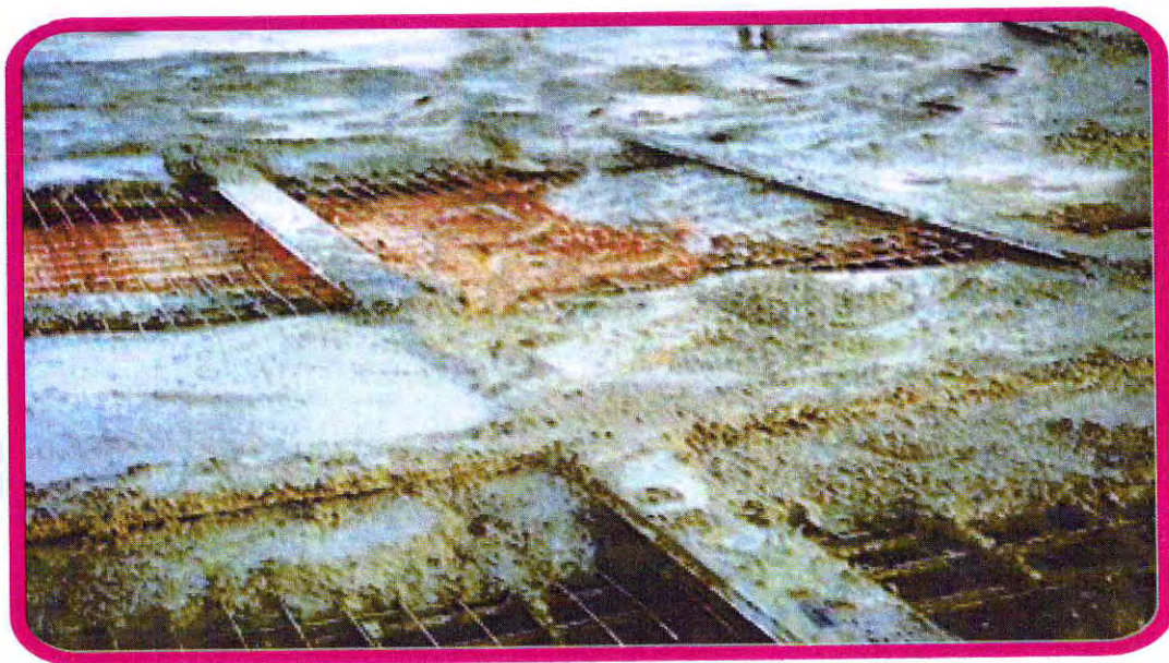
Typical in-screed type installation site
